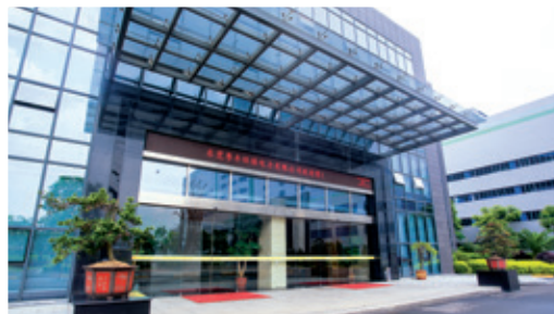
Eco-Tech II WTE Plant
