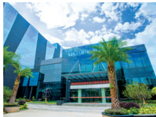
Eco-Tech I WTE Plant
